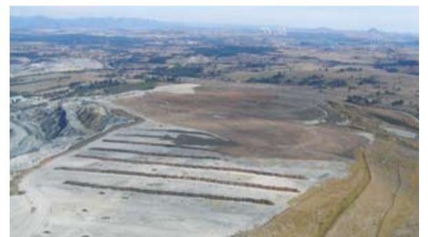
Aerial view of progressive rehabilitation works at Mt Owen.
