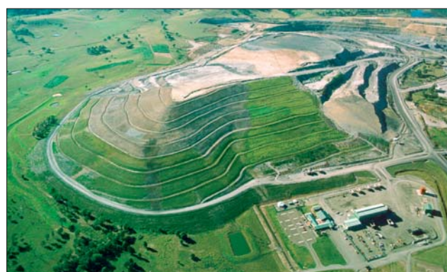
Rehabilitation is carried out in a timely manner in phase with the overall development of the mine.
